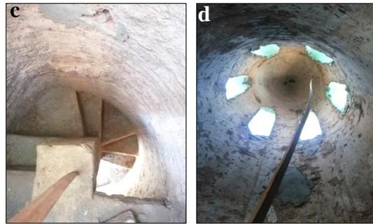
Figure (9) Shows **a.** the body of the minaret, **b.** the southeastern façade of the minaret, **c.** the stairs of the minaret, **d.** the dome of the minaret *djwasaq*.
